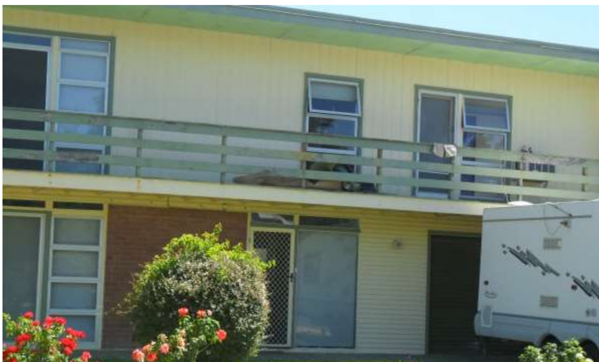
Figure 3 Photo of subject site from Bowen Street
