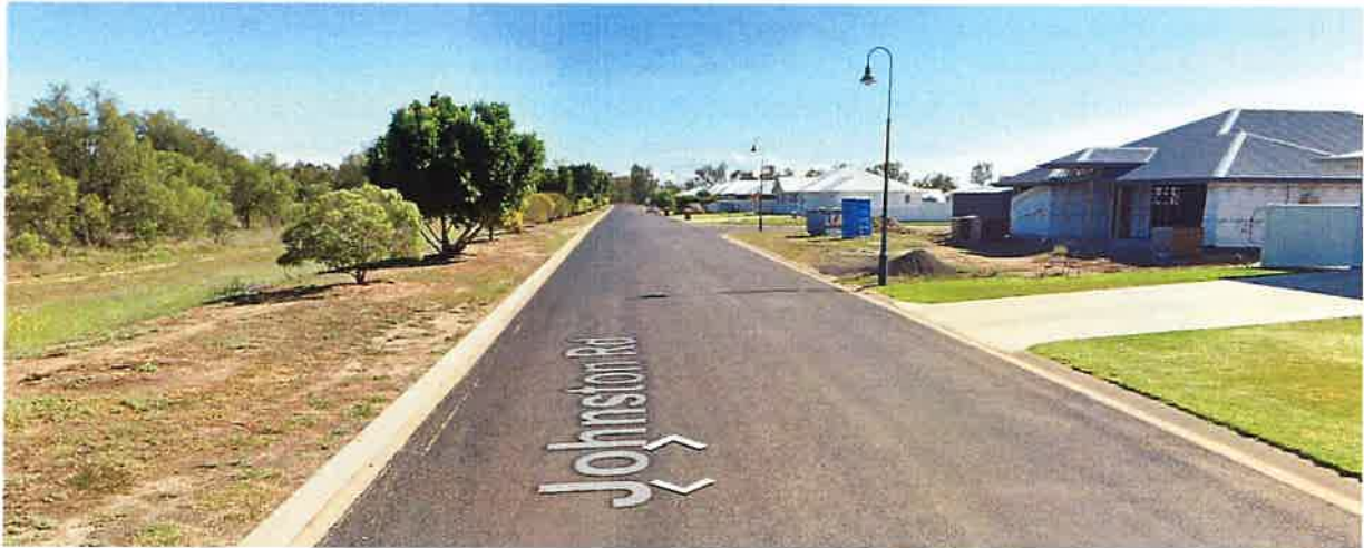
Figure 2.7 Johnston Road adjacent to Subject Site (Subject Site to the Left)
