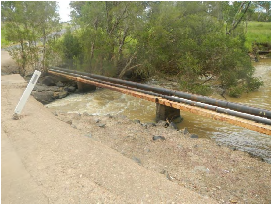
Figure 2.3 Potters Road Bridge facing downstream
