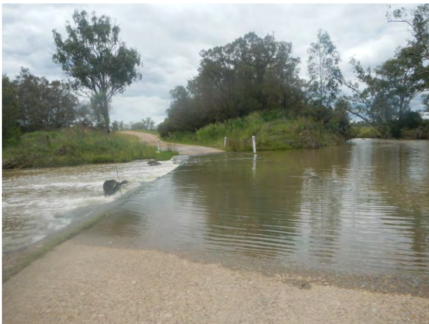
Figure 2.2 Elizabeth Street Bridge facing north
