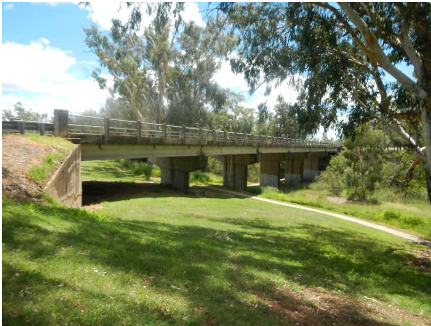
Figure 2.1 Cunning Highway Bridge facing downstream
