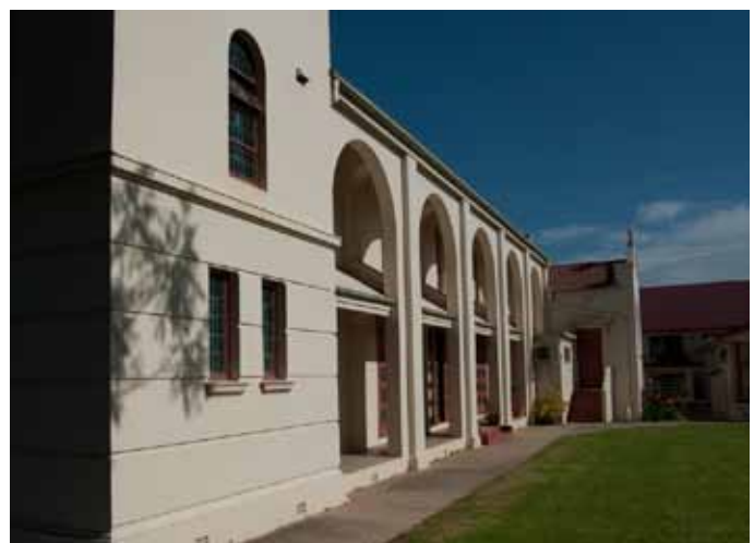
Figure 23 Arcade on eastern elevation
