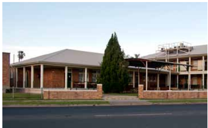
Figure 20 Goondiwindi Court House, Marshall Street
