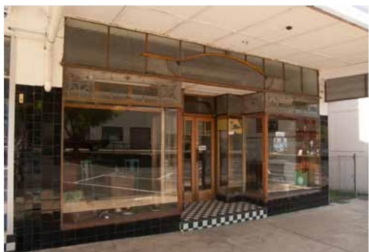
Figure 5 Shop front is highly tact with original fixtures and fittings.
