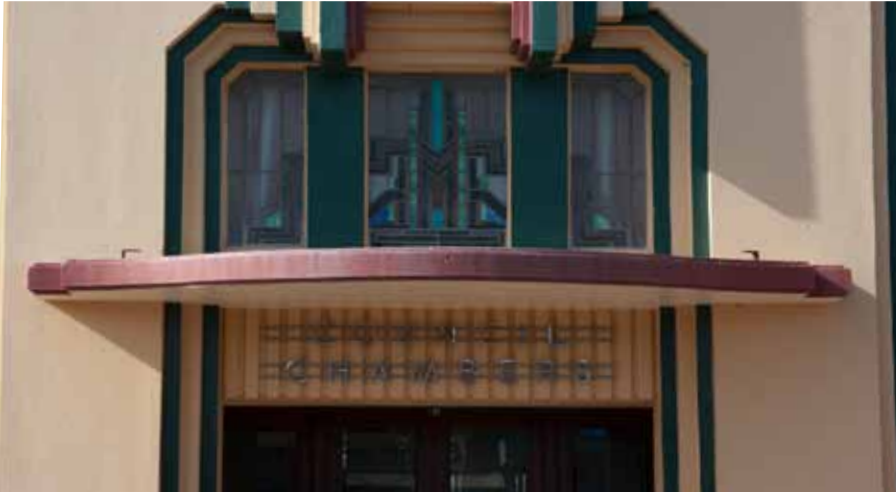
Figure 17 Awning above entrance to council chambers with lead light windows
