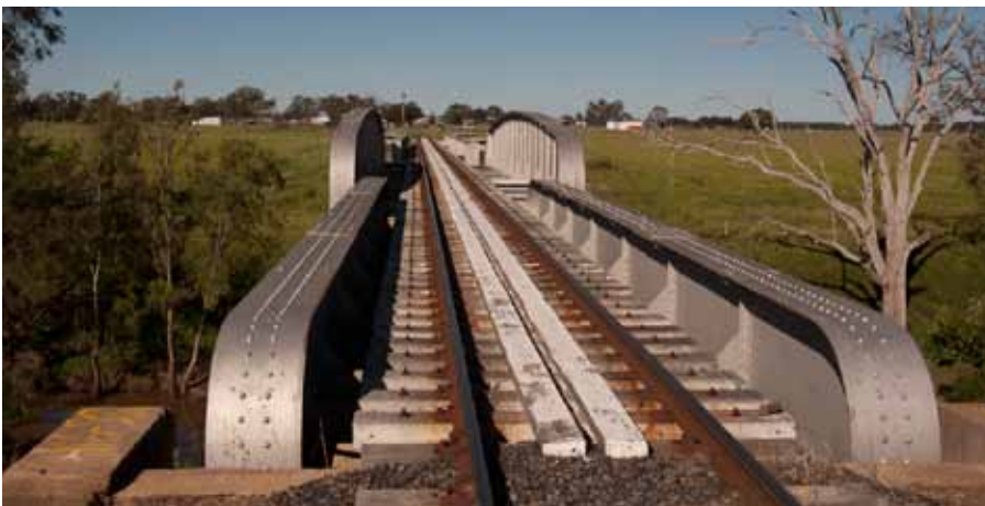
Figure 8 Macintyre Brook railway bridge, view across bridge to east
