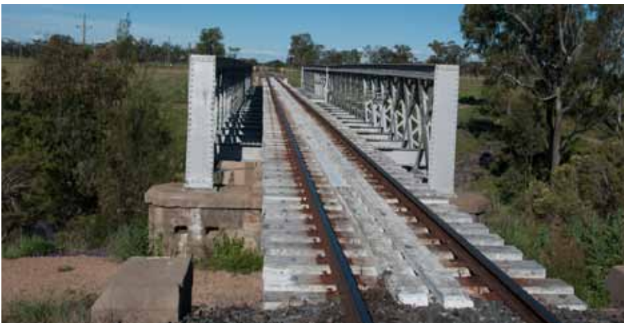
Figure 10 Railway bridge, Whetstone view to east
