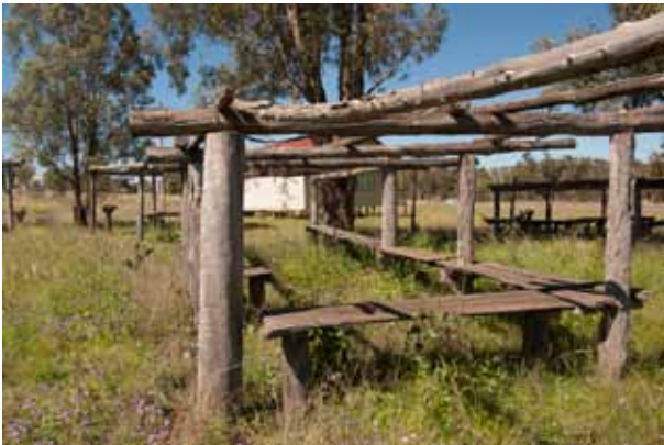
Figure 1 Shelter shed, Cement Mills recreation ground
