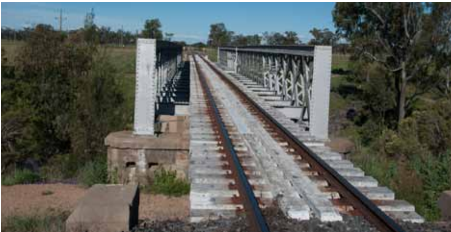
Figure 10 Railway bridge, Whetstone view to east
