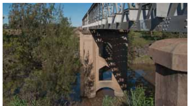
Figure 11 Concrete pier, Whetstone railway bridge
