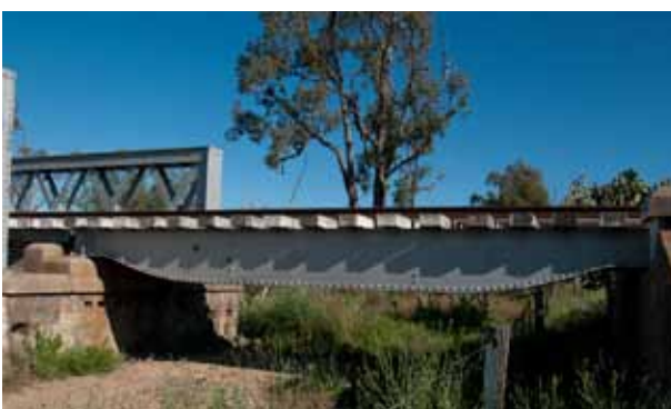
Figure 12 Fishbelly girder, western end
