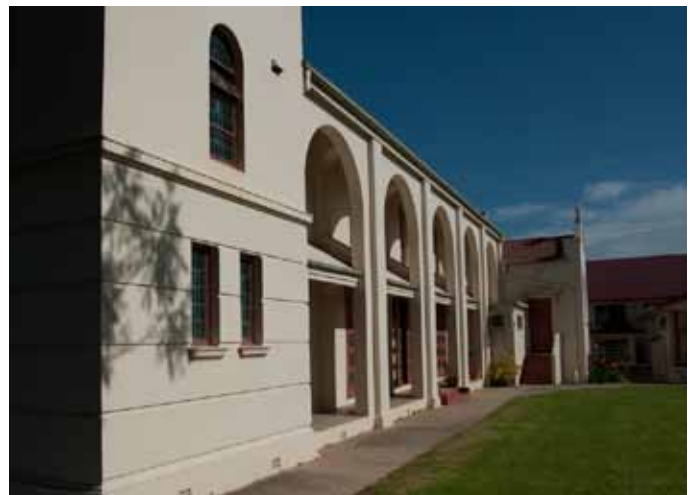
Figure 23 Arcade on eastern elevation
