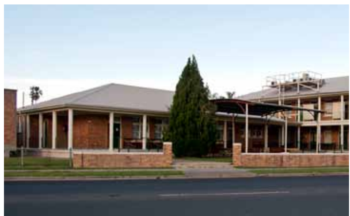
Figure 20 Goondiwindi Court House, Marshall Street
